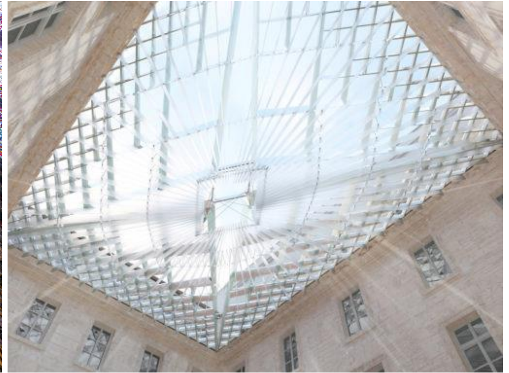
Grant for glass roof of Hotel de la Marine
